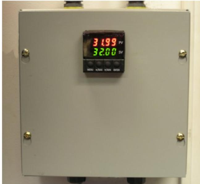
When properly connected, the Nitrox Controller will only open the oxygen control valve if the compressor is running.
